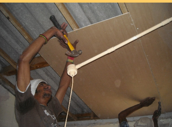
Homestay Upgrades in progress in Darling
